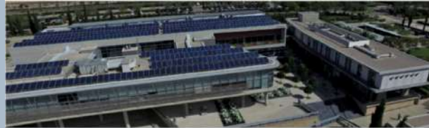
Photovoltaics within the University of Cyprus Campus
